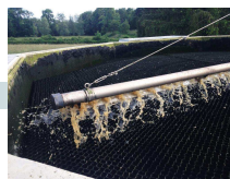
Sprinkling of inflow wastewater
