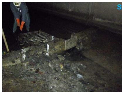
↑ Cleaning of a screen inside the sewer, March 2016
