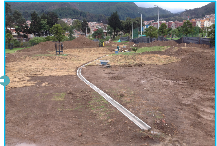
Dry extended detention basin
